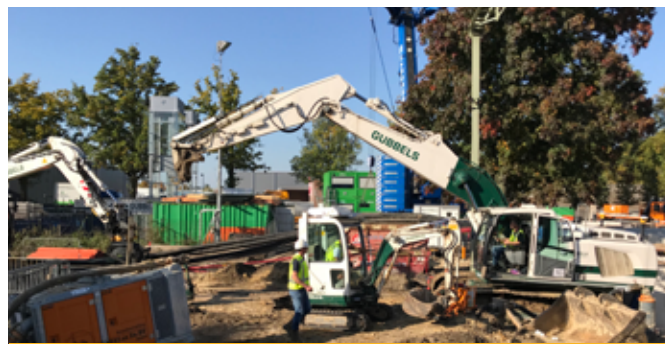
"Robuust Spoor" INFRA / BODEMSANERING
