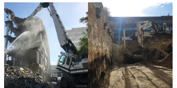
Tilburg, centrum SLOOP + INFRA
